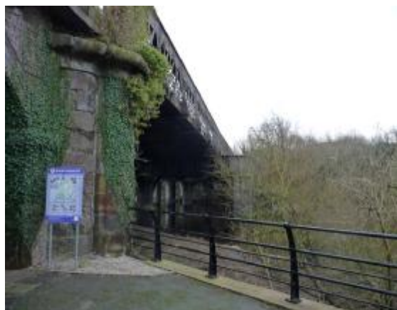
Dee railway bridge
