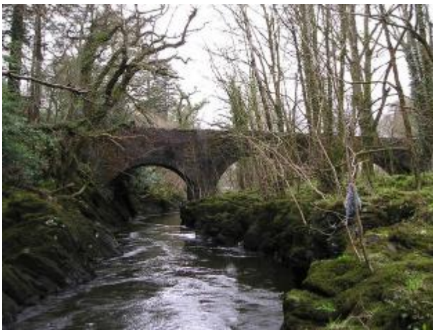
River Teifi and Henllan Bridge
